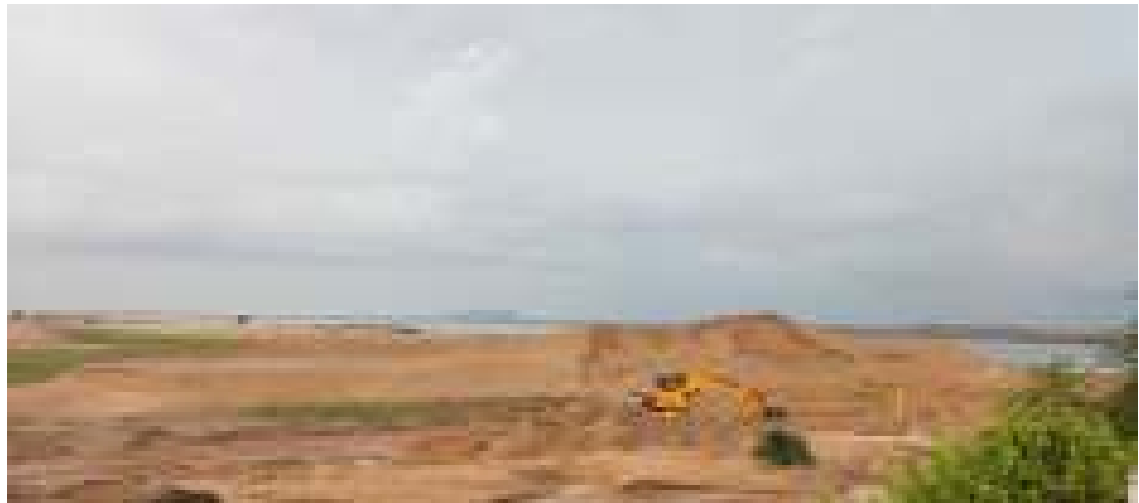
Figure 10.11 Mining of sand near Kaleshwaram along the Godavari River
